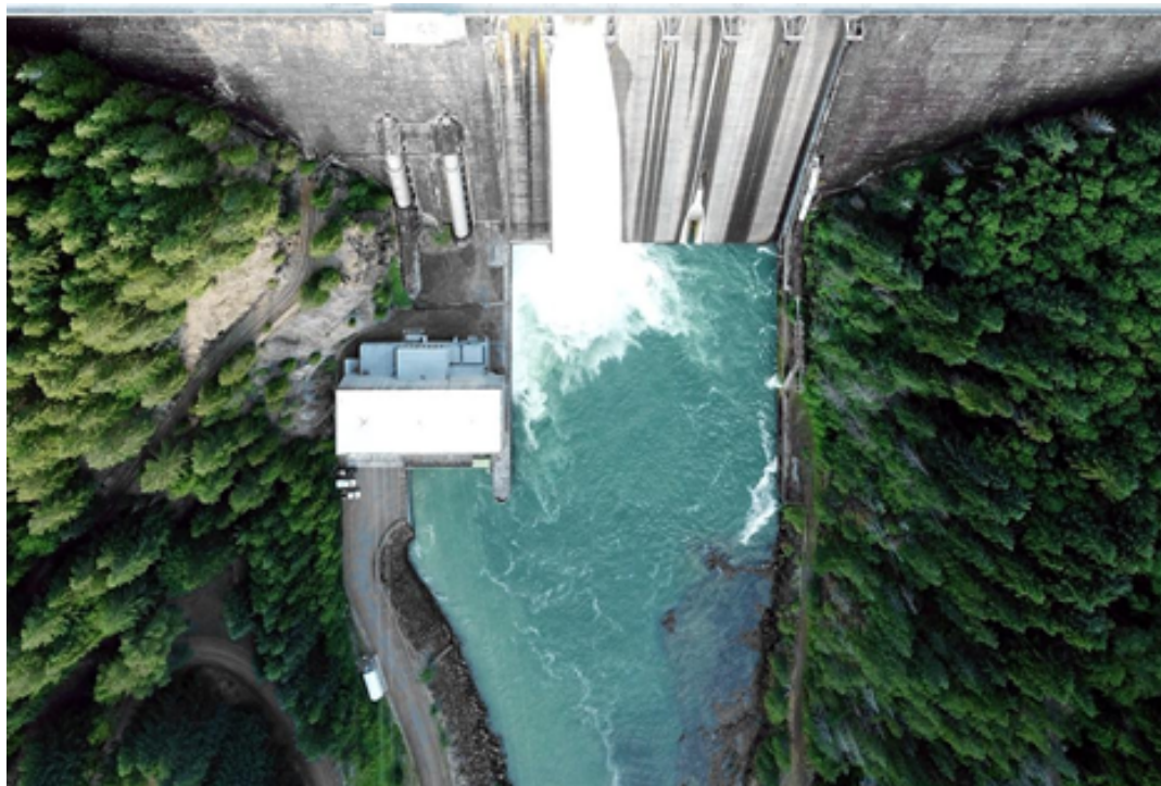
Figure 16: Detroit Dam, Detroit, Oregon, United States - Photo by Dan Meyers
