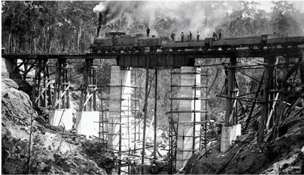
Figure 1: Bogy Creek bridge, Bairnsdale-Orbost line, circa 1914 – Photo by Museums Victoria
